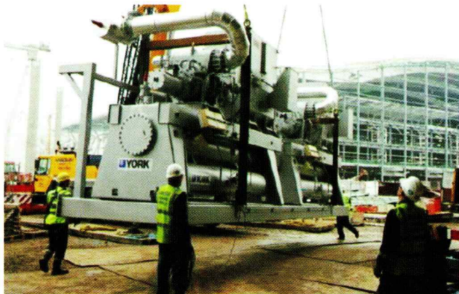
Photo 2: One of the four package ammonia chillers being installed at Heathrow airport
